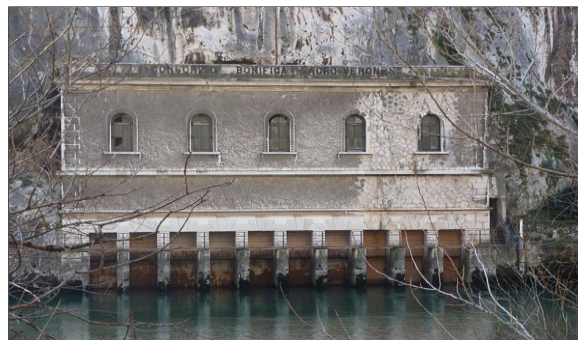
Figure 2. Chiusa di Ceraino, Rivoli Veronese, VR. Cladding system in pinkish stone, with different textures, iron frames with glass panels such as "cathedral" with blue inserts. The floodgates are made of metal rusty reddish in colour. The original floodgates were made of wood. (photo © K. Gasparini)
