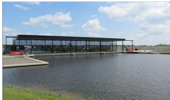
Figure 5. St German pumping station, London (photo © A.Piva)
