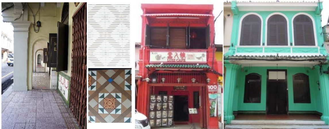
Fig.2 Veranda way & design of floor Fig.3 Rebuild or repainted outside wall of shop-houses
